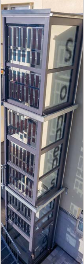
OPV module array laminated in glass façade. Please note that each module array is different
